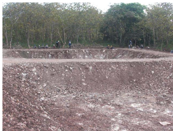
Giger East-1 Mud Pit Construction
