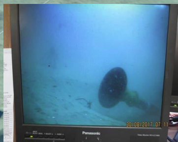
Completed umbilical bell mouth on sea bed
