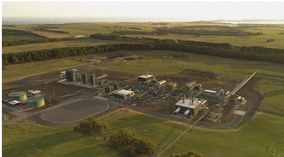
Athena Gas Plant
