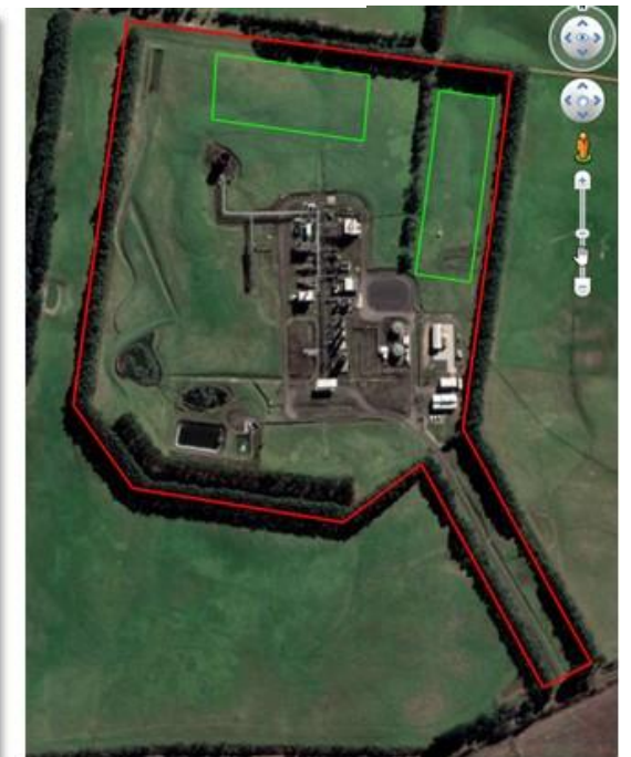
Athena Gas Plant showing conceptual footprint of 2 x 2.4MW solar arrays
